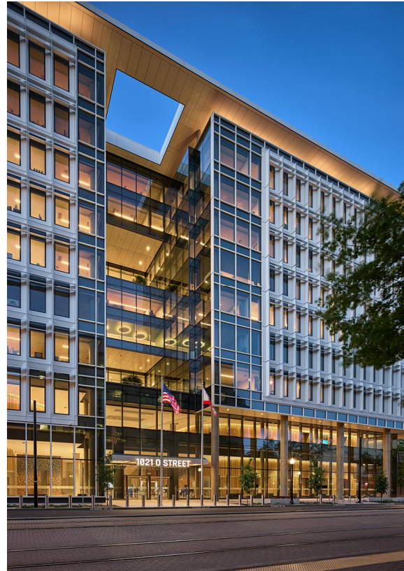
DGS 10 th & O Street Sacramento, CA 478,000 SF LEED Platinum | Offsite dedicated solar PV | Carbon Neutral
