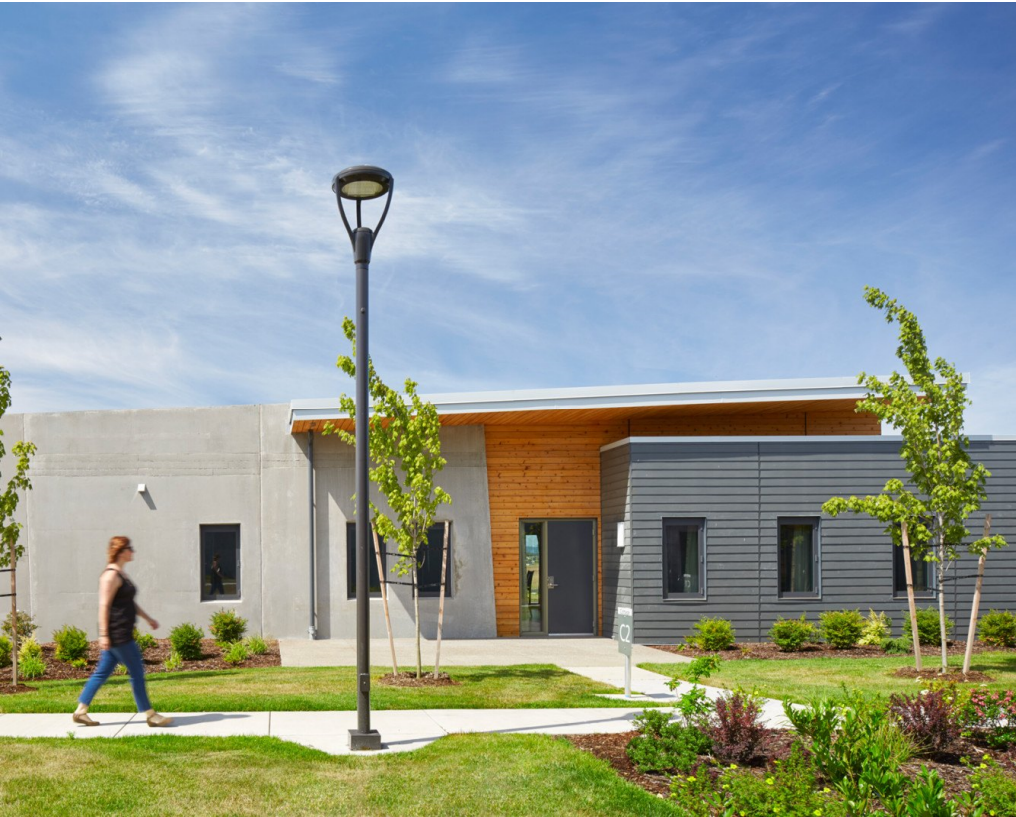
Oregon State Hospital Junction City, OR 220,000 SF, 174 beds Geo-exchange + Onsite solar PV | Carbon Neutral
