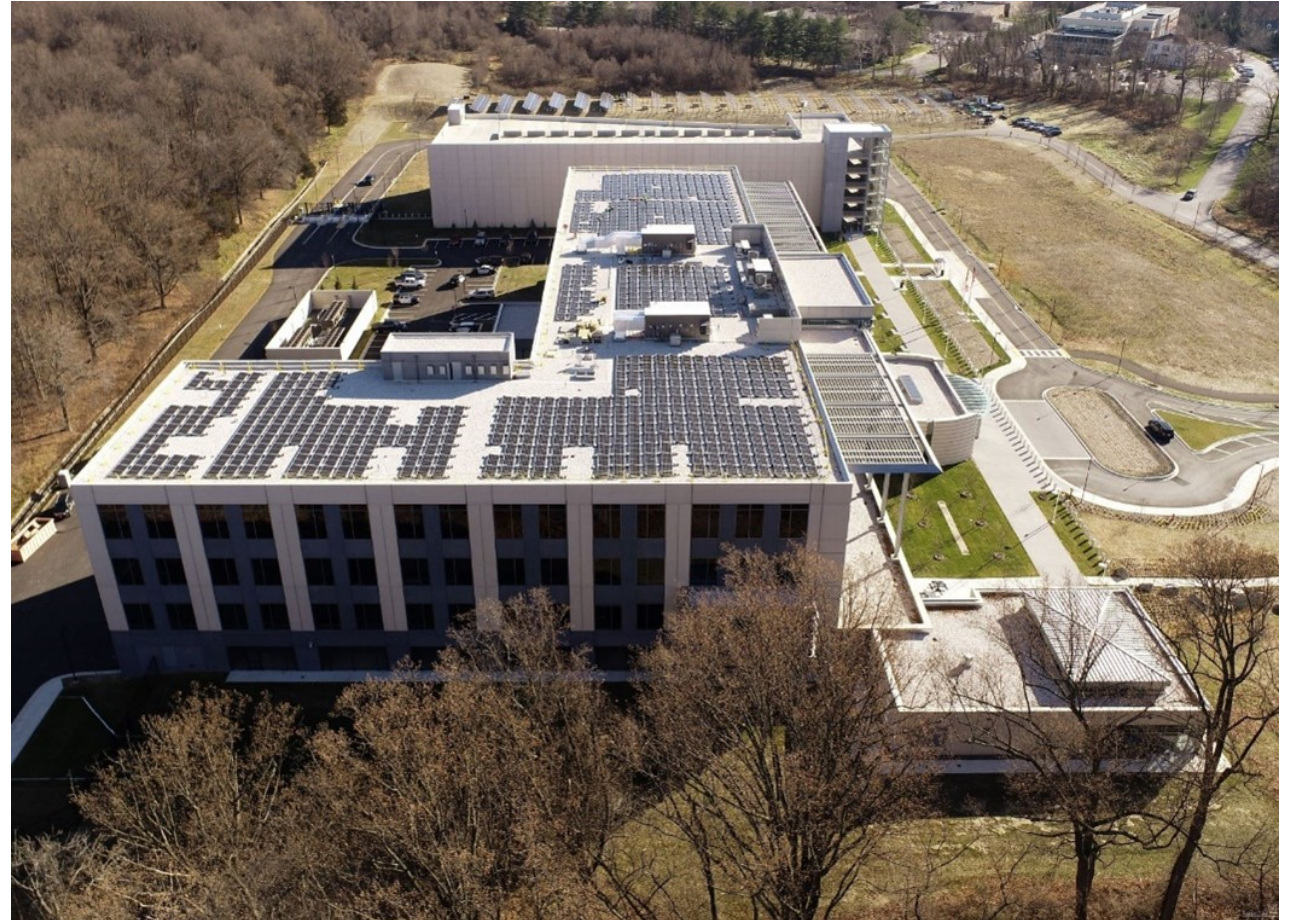
Howard County Circuit Courthouse Ellicott City, MD 238,000 SF, 12 courtrooms LEED Gold | 60% onsite generation + offsite generation
