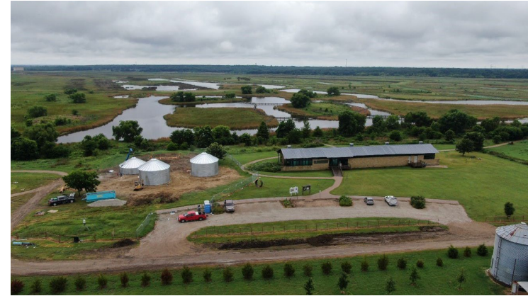
NTMWD East Fork Water Reuse Project Wetland Education Center (Texas)
